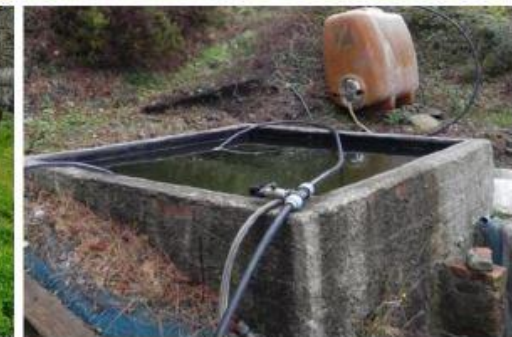
Fig. 2. The typical concrete tanks, used for traditional irrigation in the CTNP.
